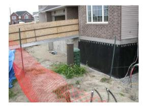
A catwalk from the street to the main entrance of the residence is erected. In fact, the excavation looks a little like a rabbit warren once all of the soil from around all of the foundation is removed. Houses stand without
