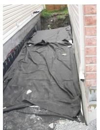
Landscape cloth is used to keep fill from subsiding into cracks, prior to backfilling and finishing of the landscape.
