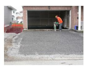
The lightweight fill is then topped with topsoil, and driveways, planting, sod, etc. is installed. Garages and driveway areas are capped with granulars to provide for proper slope and finished as per specifications and requirements.
