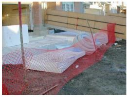
It is important to note that the weeping tile system is installed at the perimeter of the lightweight fill and not around the perimeter of the foundation. The weepers are then connected to the previously existing drains.
