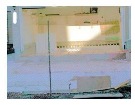
If leveling is required (note that the home usually rebounds significantly (20 mm) when soil loads are removed from around the foundation), brackets are installed on the foundation and the foundation is reinforced (typically straps fastened / bonded to the top and bottom of the wall). Jacks are then placed on the brackets and the foundation wall is jacked off the footing until level. The next photos show the "before" and "after" of this process.
